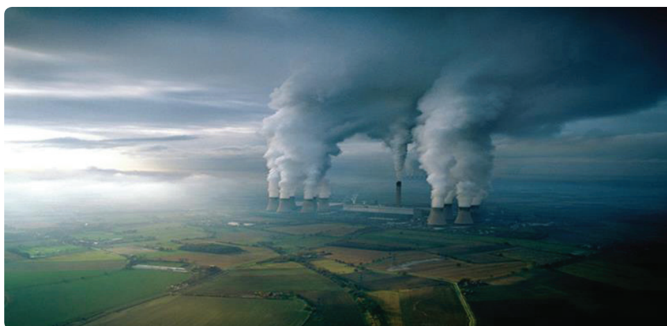
Figure 2: Shows a photo of the cooling tower: https://acs-nnov.ru/gradimi-tec.html . Under the normal load of the CHP, one-unit cools over 10,000 cubic meters of liquid per hour. Artificial evaporations from cooling towers begin to prevail over organic ones.
